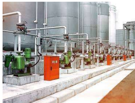
Self-priming type pumps in a paint manufacturing plant.
