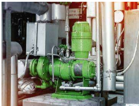
High-temperature type pump in a chemical plant.
