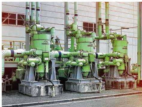
Reverse circulation type pumps for pumping LNG as Cooling medium. (Vertical type, Motor output 75kw)
